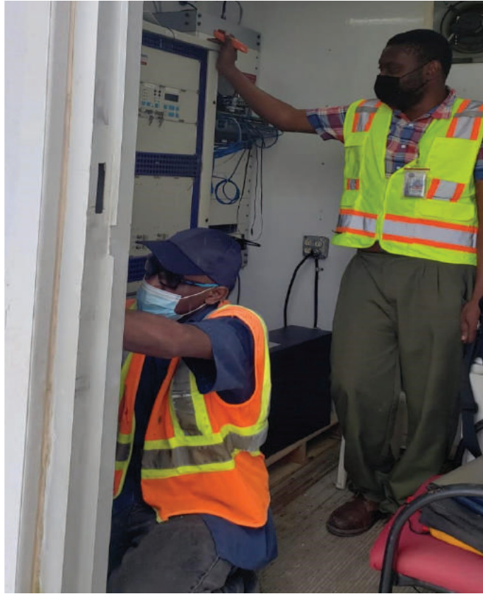
Installation of transducers at the NMIA Instrument Landing System (ILS) site by members of the electrical team.
